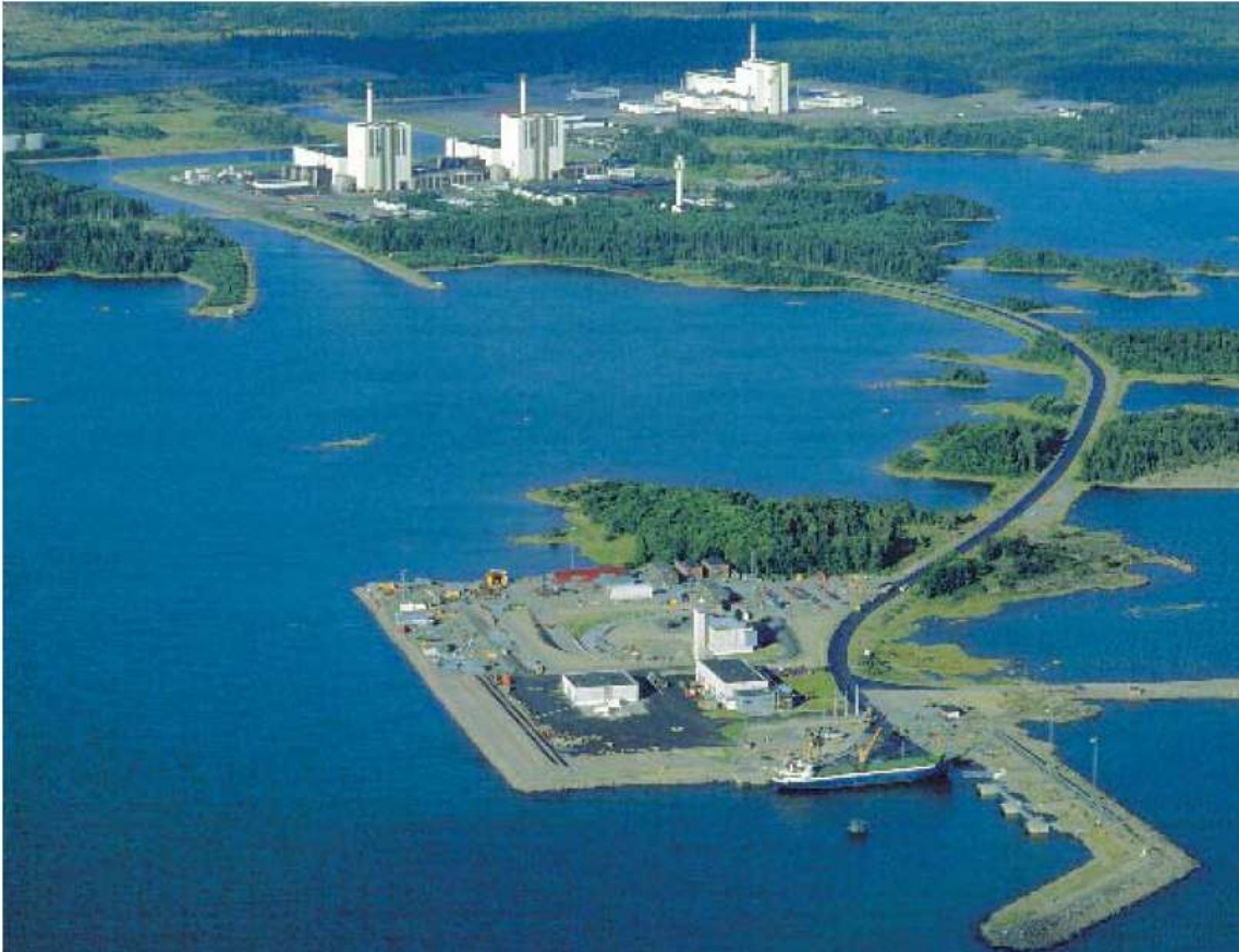
Figure 7.1. SFR receiving station and the three reactor blocks of Forsmark in the distance.
