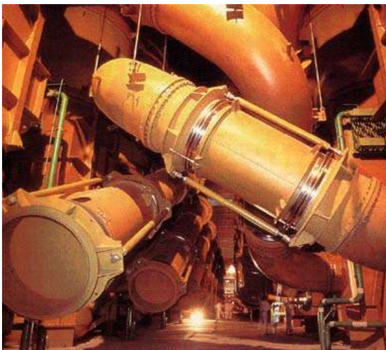
Figure 4.1. Tubing and filters for \text{UF}_6 enrichment.
